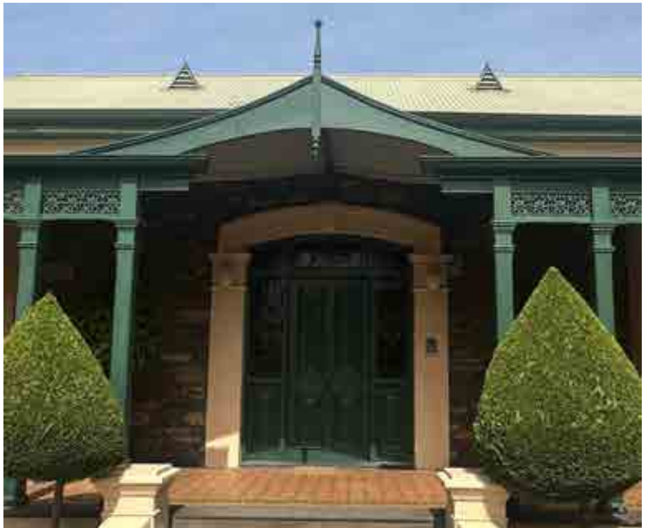
Figure 10: 1980s reproduction verandah detailing on 99 Palmer Place
