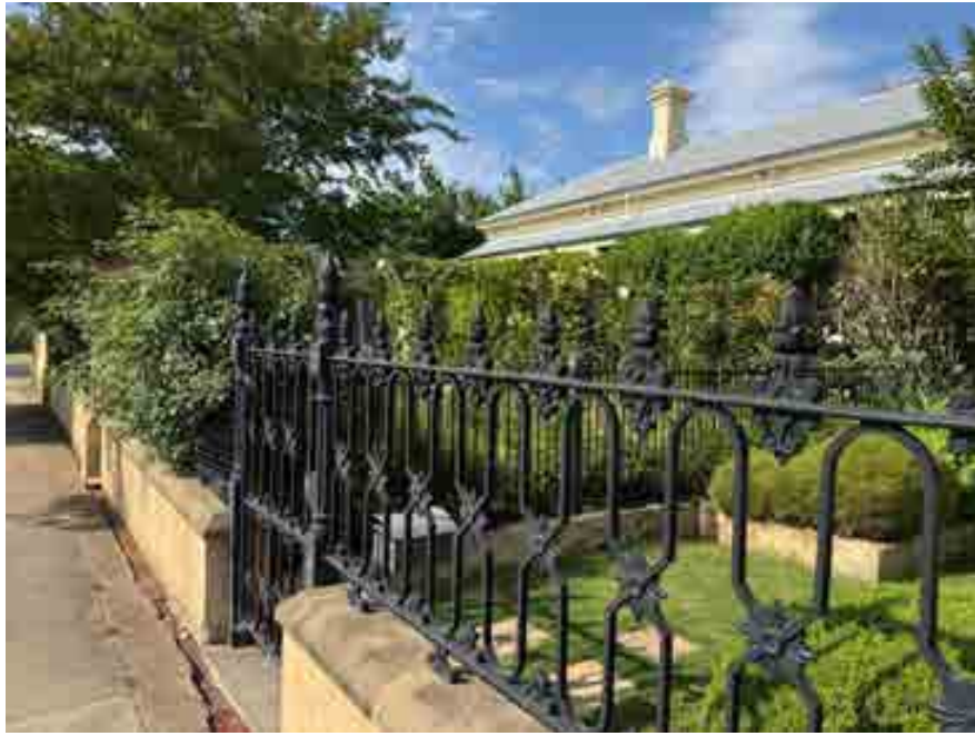
View North – 84 Mills Terrace: Predominant Character Returned
