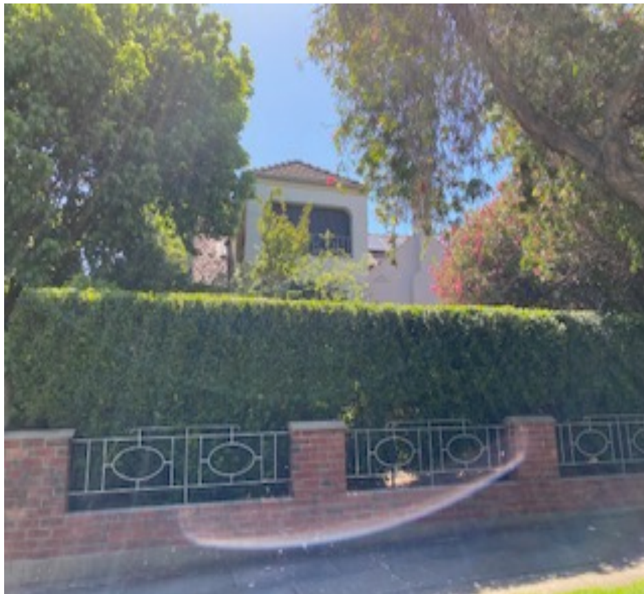
66, Mills Terrace: The Subject Property
